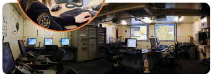
Panoramic view of Shelter's interior
